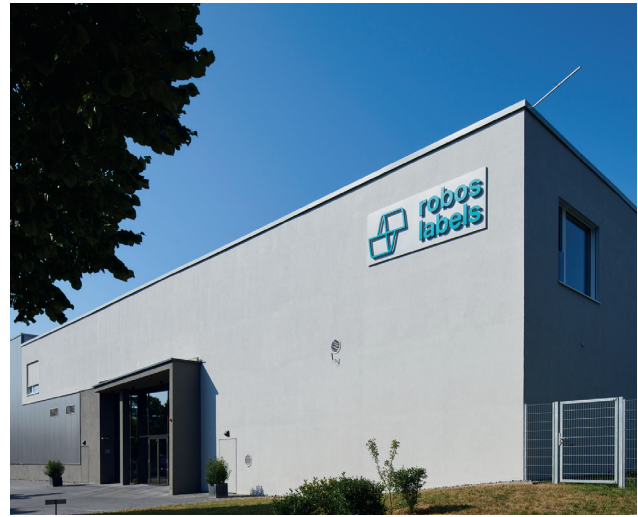
Our Headquarters in Kornwestheim - Administration and Manufacturing
