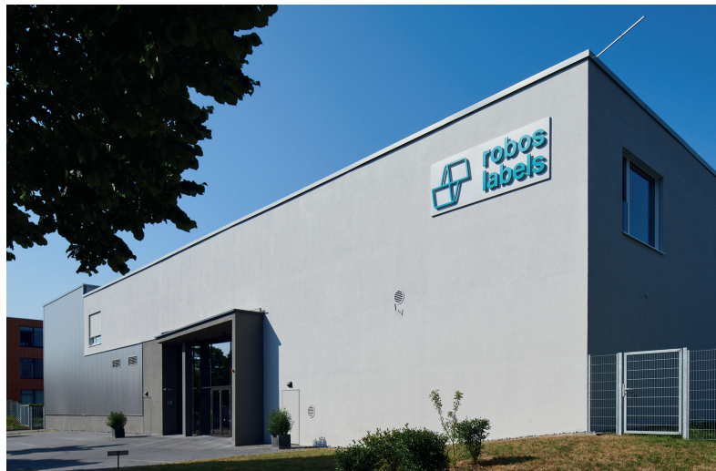
Our Moldengraben Site Combines Administration and Production.
