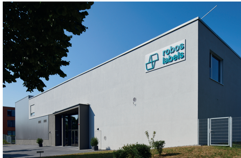
Our Moldengraben Site Combines Administration and Production
